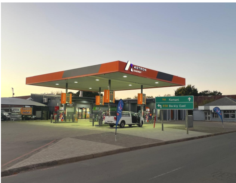
PHOTO: ASTRON ENERGY ALIWAL NORTH.
